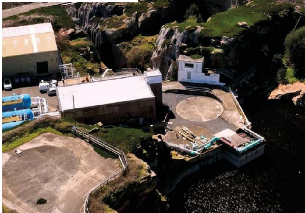
The desalination plant. Photos credit: Max Burnett
