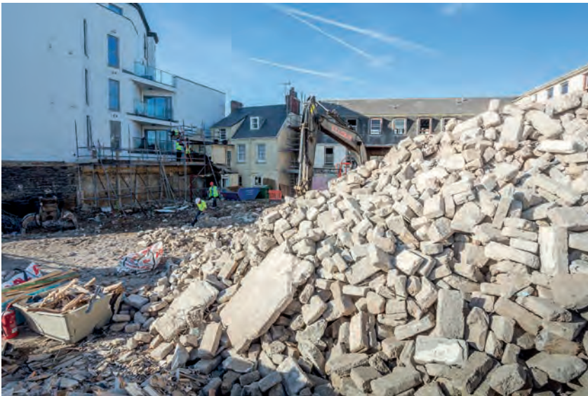
Segregated waste sourced from the demolished Fort d'Auvergne Hotel.
