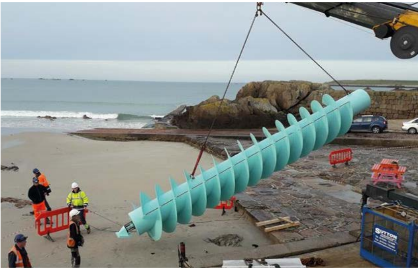
Left: One of the Archimedes pump screws, being installed at Le Dicq in June 2019. Right: Part of the Canal as shown on the 1795 Richmond map
